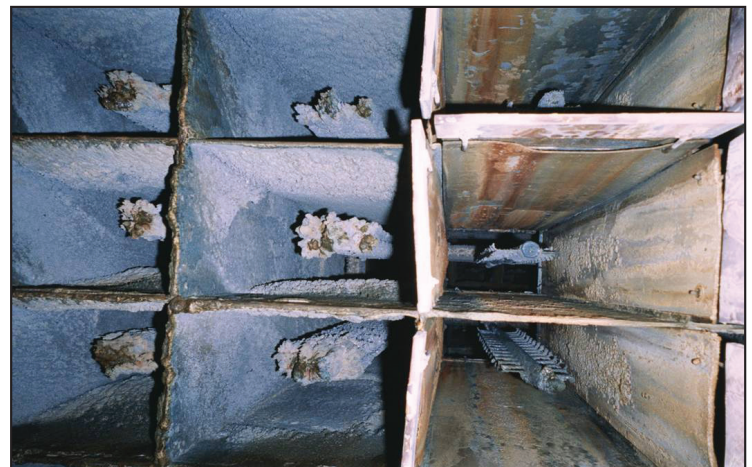
DIRTY METAL PLATES (INTERMITTENTLY CLEANED DURING OPERATION)
