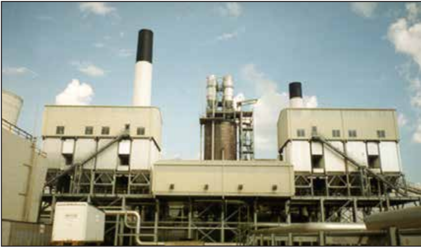
Fabric Filter Removing Particulate From 4 Coal Fired Boilers – 780,000 lb/hr Steam Total
